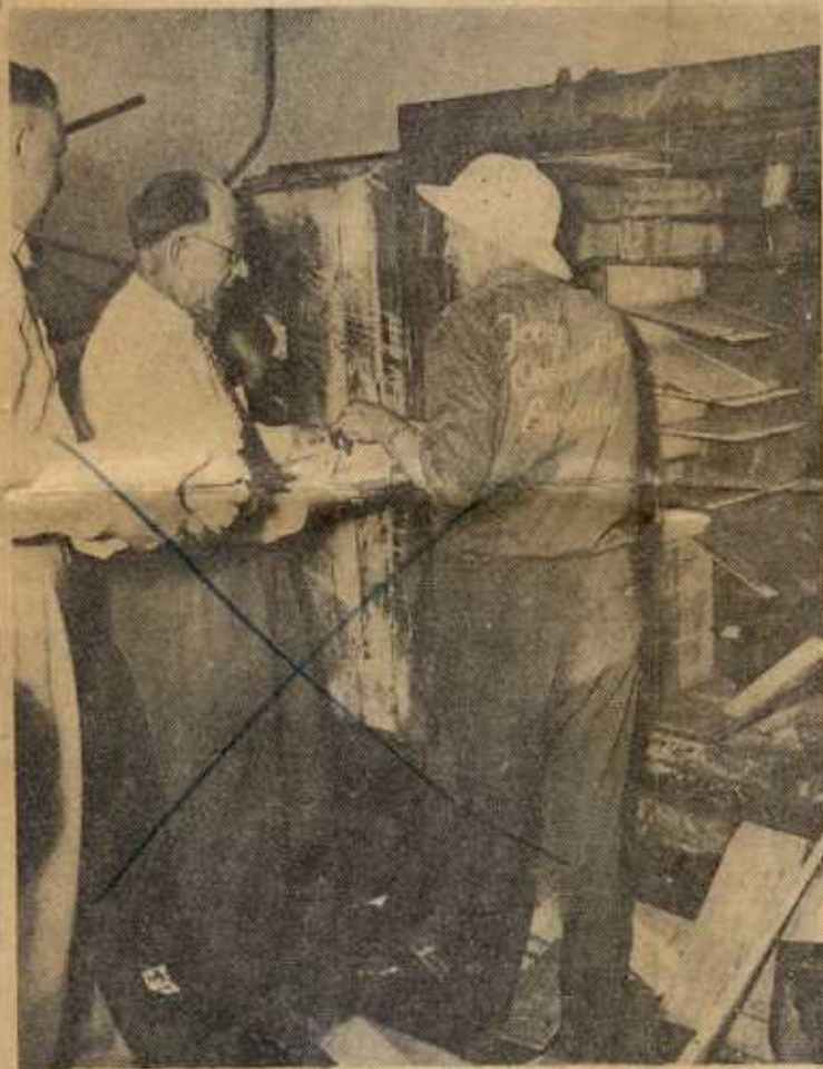
SAFE RECOVERED IN FIRE RUINS —Stanley T. Anderson, center, general manager of the fire-destroyed Alliance Furniture Company plant in Allen Street, is shown examining records taken from a safe recovered from the ruins. The safe was opened by Jerry Okerlund, contractor, shown at right. Assistant Fire Chief Bernard Swanson is shown at left. The safe contained all company records, some $600 in cash, and $80,000 in invoices. The records were intact, although damaged by water and fumes.
